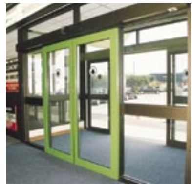
Location: Guernsey Airport Architect: Patrick Reade, States Architect Fabricator: Window Design Ltd
