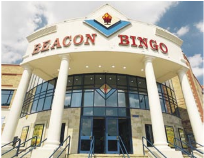
Location: Beacon Bingo, Cricklewood Architect: John Sisk & Sons Fabricator: Fox Aluminium Services.
